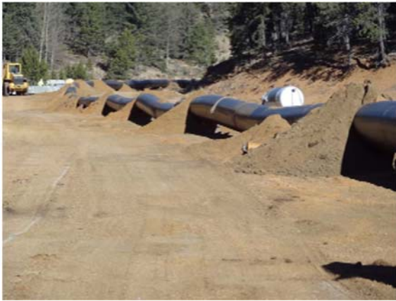
Uphill from launch site pipe staged
