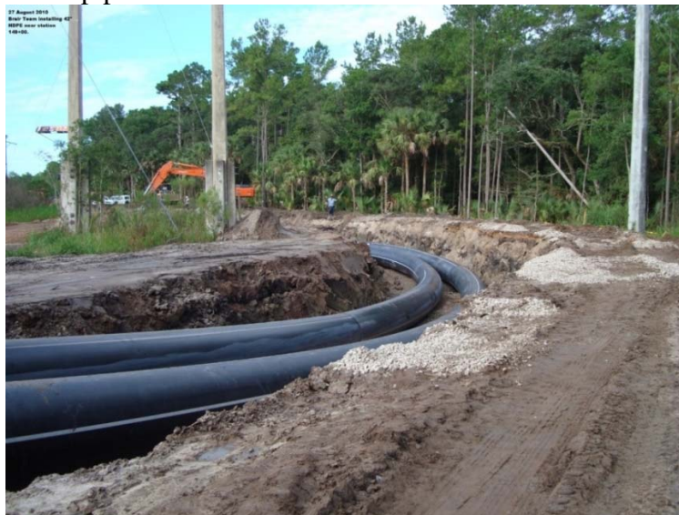
Figure D.2.7 Photograph of challenging bend
