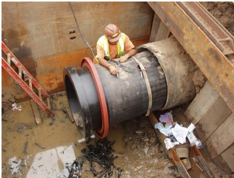
Figure D.1.3 Access pit to the steel host pipe
