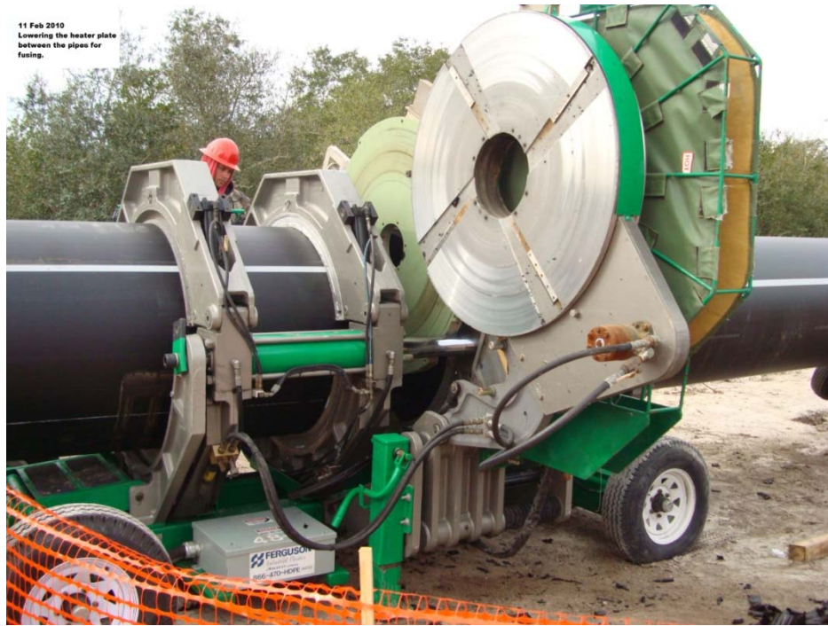
Figure D.2.5 Lowering the heater plate between the pipes for fusing
