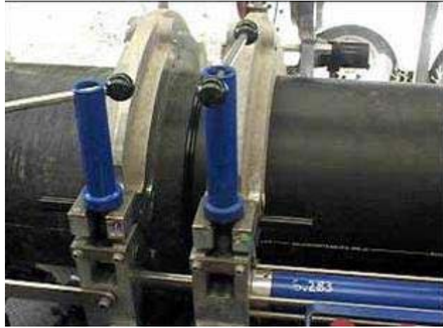
Figure D.4.1 Joints were butt-fused for the MDT pipeline project
