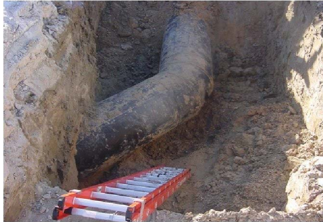
Figure 6.6 45-deg bend used in the Houston pilot study
