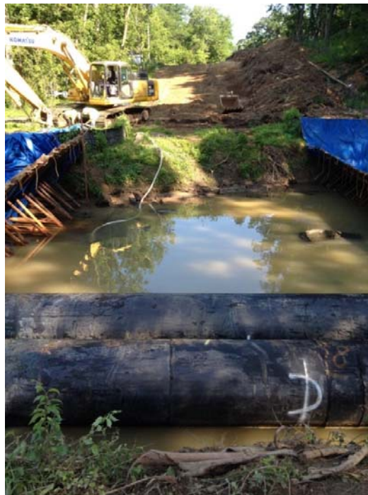
Figure D.10.2 The project involved one river crossing
