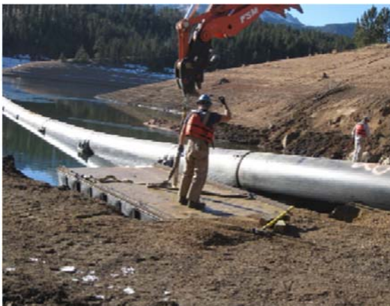
Ballasts attachment area
