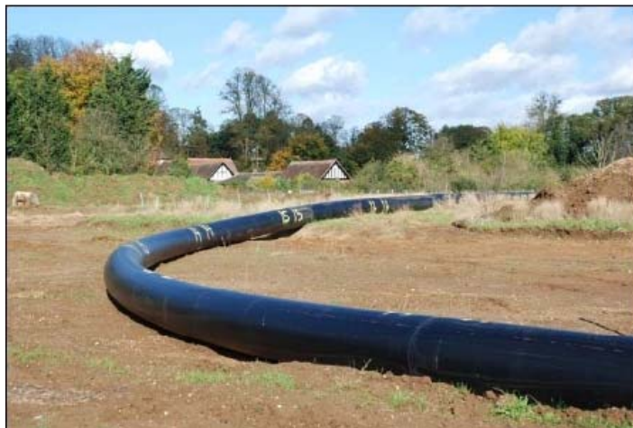
Figure 6.9 A view of the Gatehampton Bore Hole project site during installation
