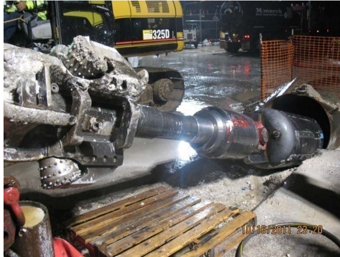
Figure D.8.2 Pulling of HDPE pipe following drill and reaming operations
