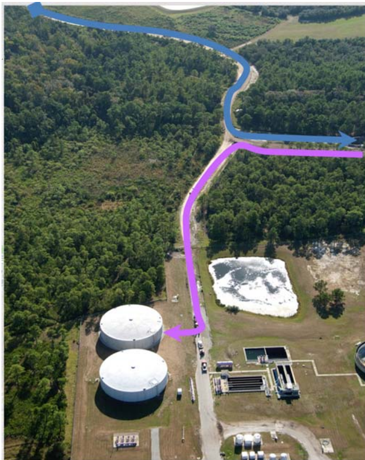
Figure D.2.1 Finished reclaimed water to ground storage tanks (Purple), raw water pipeline route from RWPS (Blue)
