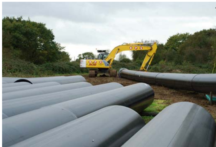
Figure D.9.1 A view from the construction site
