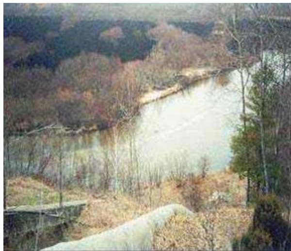
Figure D.4.3 The 30-mile long was installed along a challenging terrain
