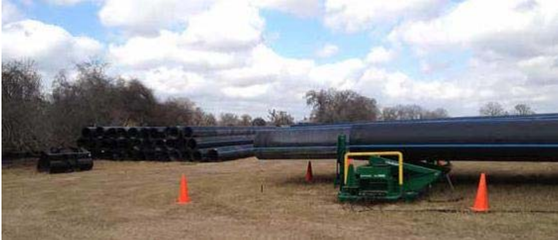
Figure 6.8 HDPE pipe segments stacked in field prior to installation
