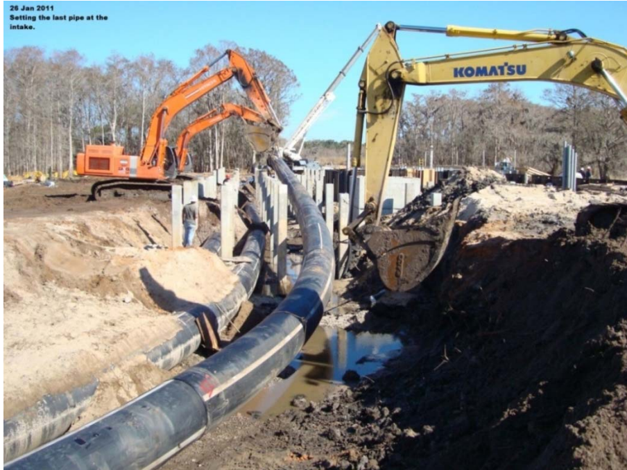
Figure D.2.8 Final pipe bend and tie-in
