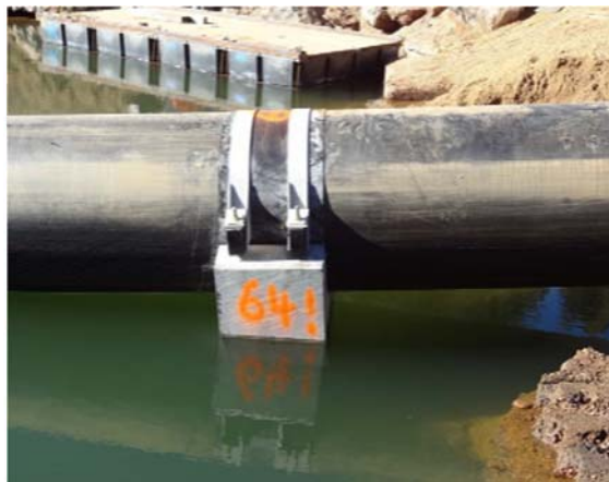
Ballast attached ready to launch
