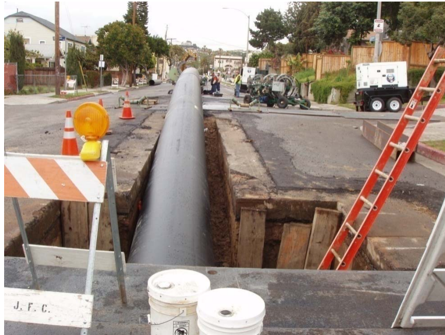
Figure D.1.1 The 36 in. HDPE being inserted into the host pipe
